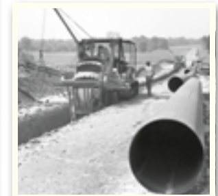
▲ Pipeline construction, 1960s.
