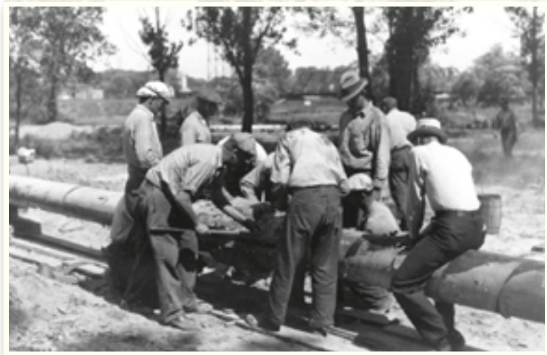
▲ Gas pipeline construction, 1931.
