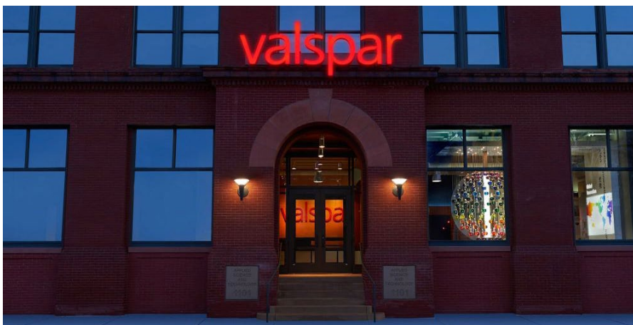
Valspar Applied Science Technology Center and Headquarters Building, Minneapolis, MN.
